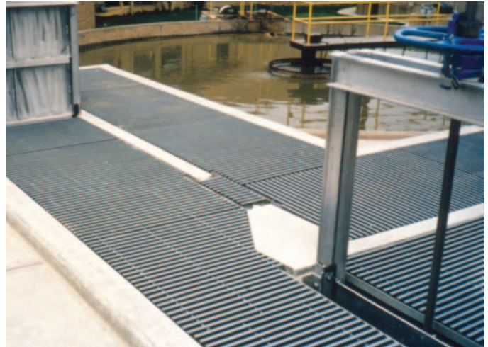
Low maintenance fiberglass grating provides trouble free operations for the covers and walkways in the Lakewood, Colorado Wastewater Treatment Plant Headworks. DURADEK® I-6000 1-1/2" was used.
