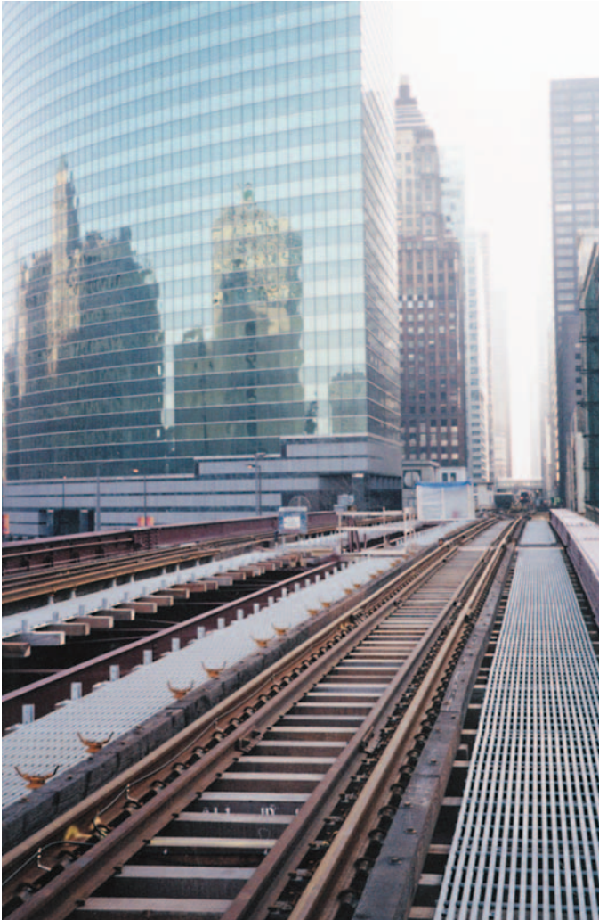
Chicago Transit maintenance walkways alongside elevated train tracks constitute one of the largest fiberglass grating installations in history. This project used DURAGRID® T-5000 2" with a custom polyester resin.
