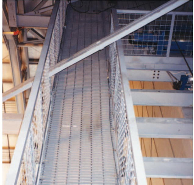
DURAGRID® I-7000 1-1/2" provided lightweight (70% open space) platforms for the Fedex 747 hanger at the Anchorage, Alaska Airport.
