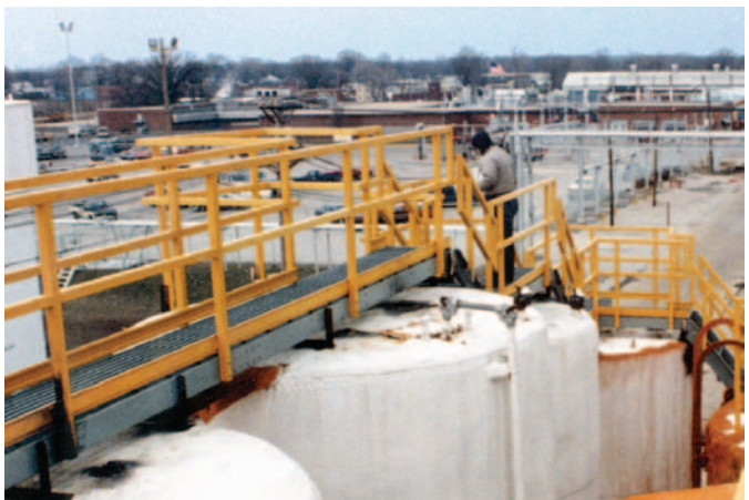
A heavy duty handrail system that uses 2" x 1/4" EXTREN® square tube built to ASTM F-1092-87 specifications is available for applications requiring added stiffness for less deflection under normal loading.
