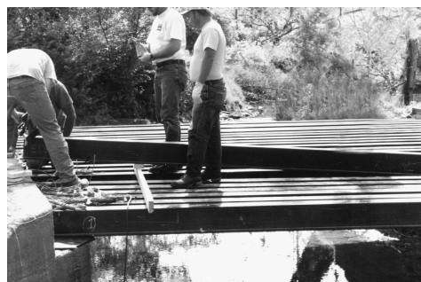
Figure 30. Installation of the Tom's Creek Bridge.
