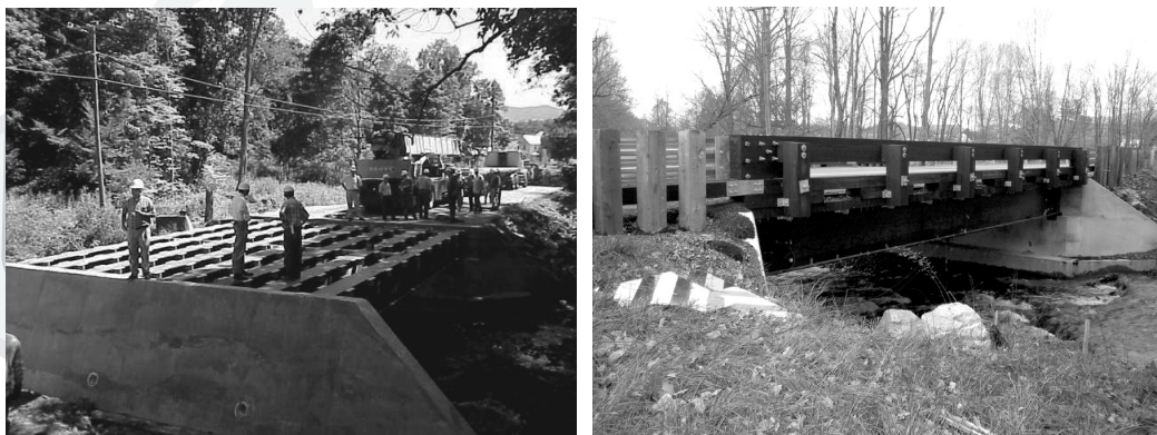
Figure 31. Route 601 Bridge Superstructure
